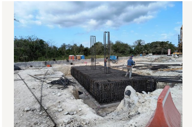
Assembly of foundation reinforcement.
